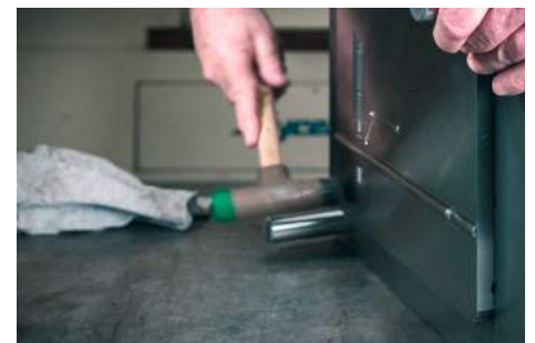
Installing the insert
